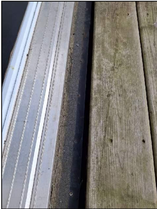
8. Missing flashing
