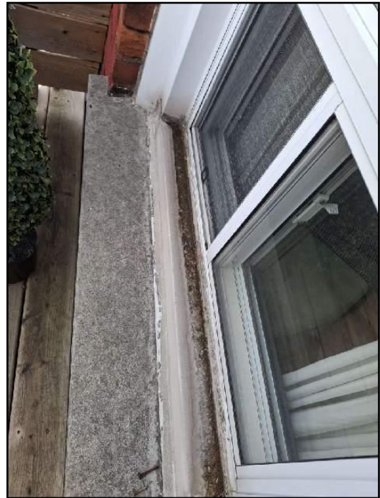
9. Poor slope
