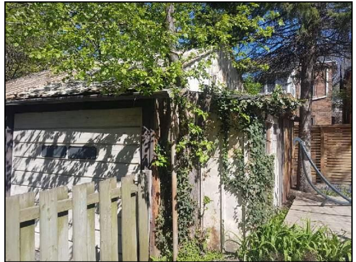
10. Typical low quality structure
