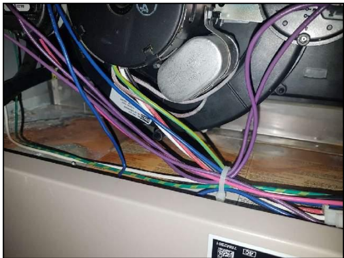
10. Condensate leak
