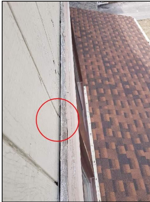
1. Caulking missing or deteriorated
