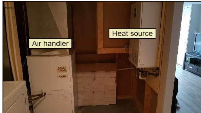
3. Combination heating system
