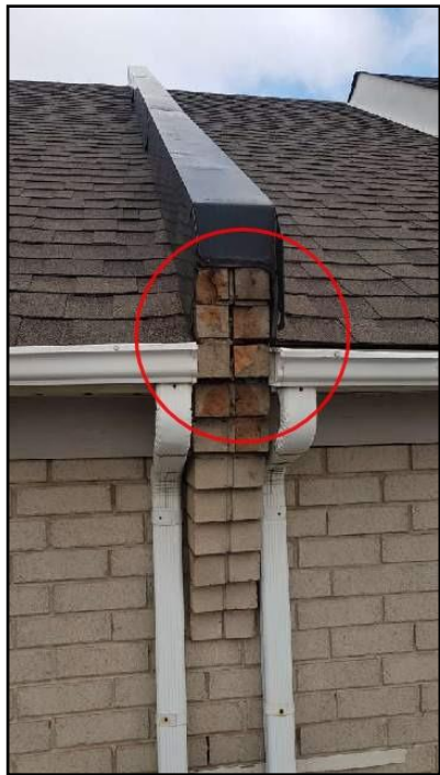
1. Spalling
