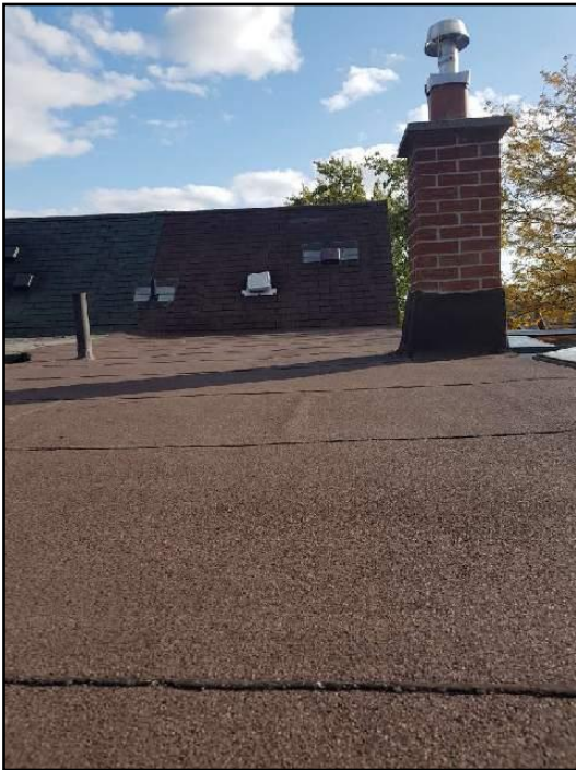
2. Modified bitumen membrane
