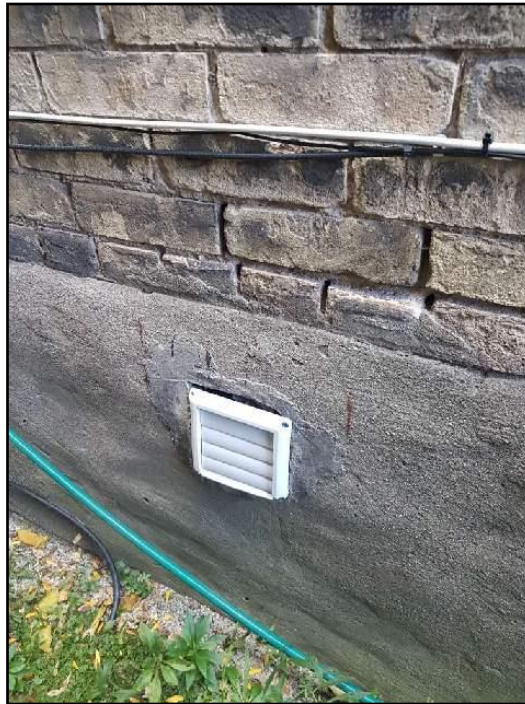
6. Seal vent at wall
