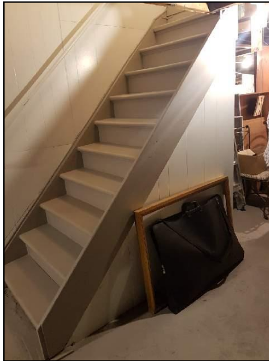
18. Missing guardrail
