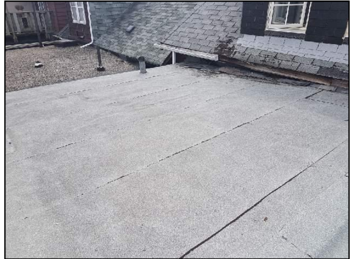
2. Modified bitumen membrane
