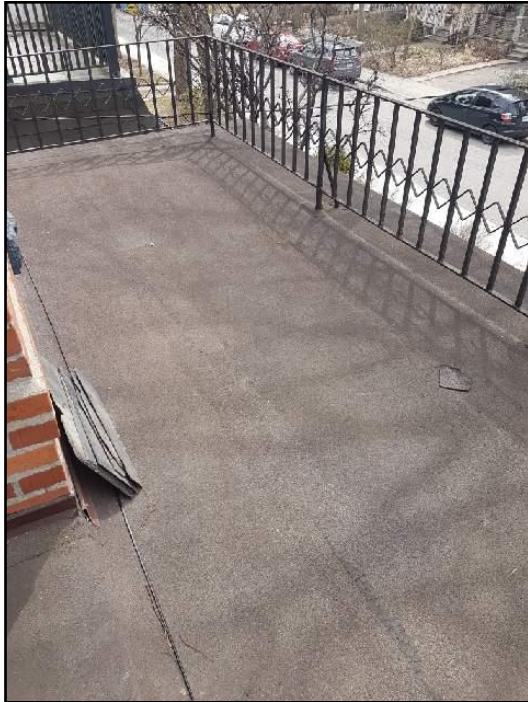
1. Modified bitumen membrane
