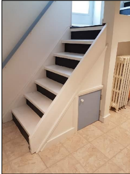
5. Missing Guardrail
