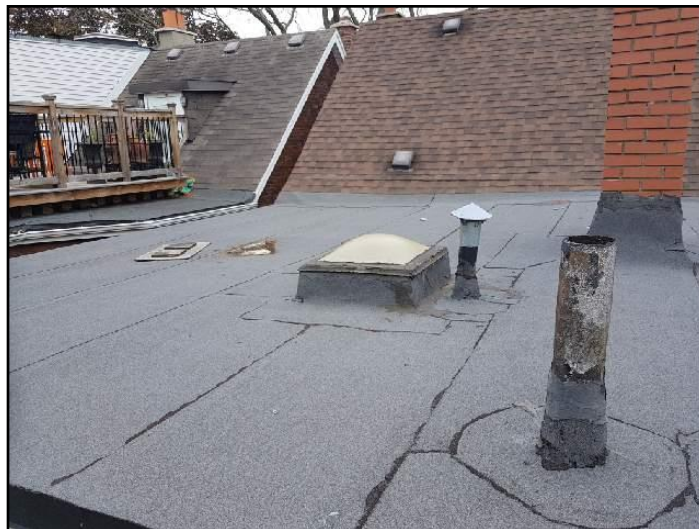
2. Modified bitumen membrane
