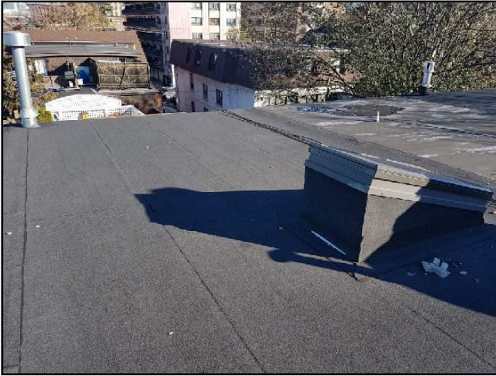
3. Modified bitumen membrane
