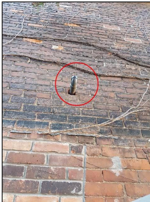
13. Poor vent pipe arrangements
