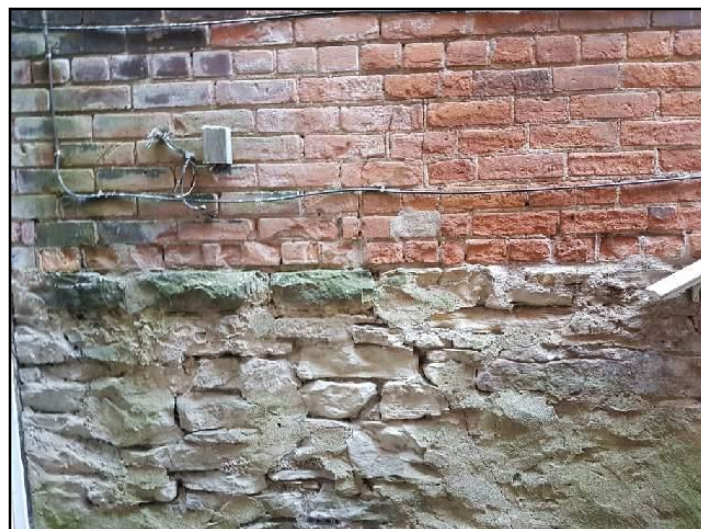
7. Parging damaged or missing
