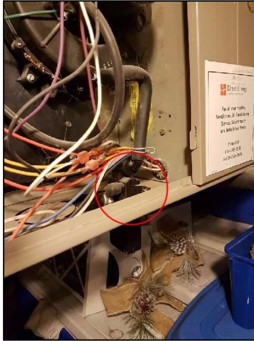
12. Condensate leak
