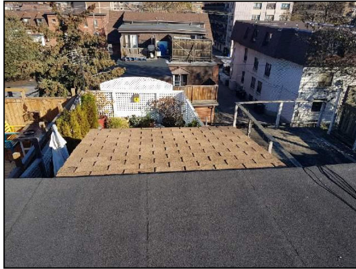
1. Asphalt shingles
