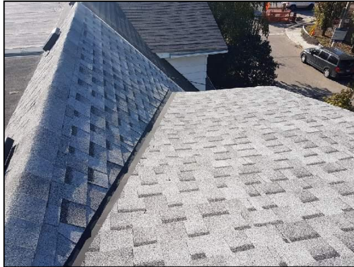
1. Asphalt shingles
