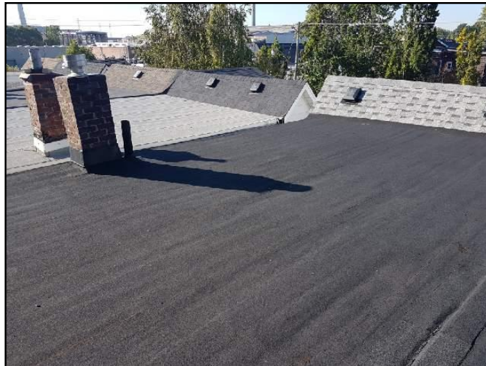
2. Modified bitumen membrane
