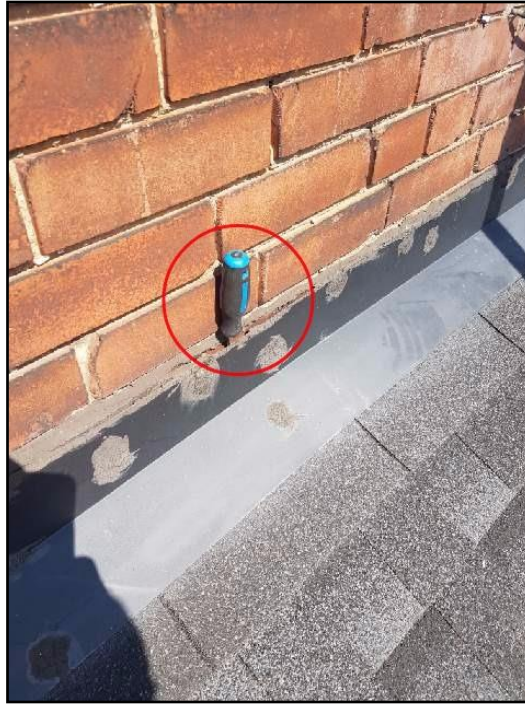
3. Loose flashing
