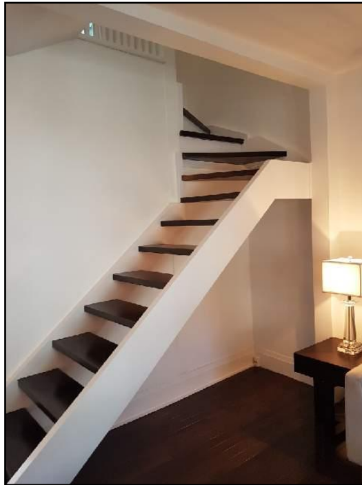
15. Missing guardrail
