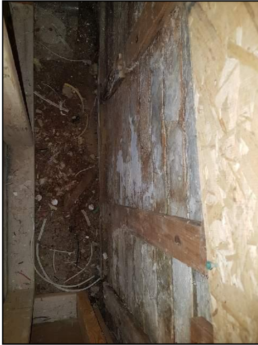
16. Dampness on floor or walls
