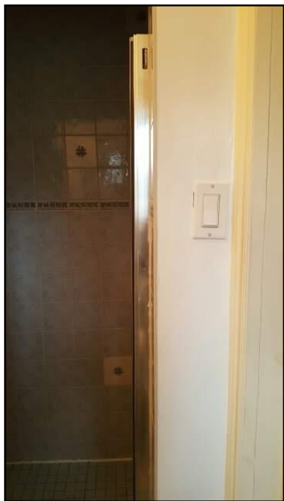
10. Location poor (near Bath Tub or Shower Stall)
