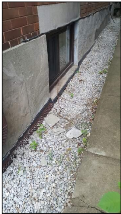
25. Recent exterior excavation
