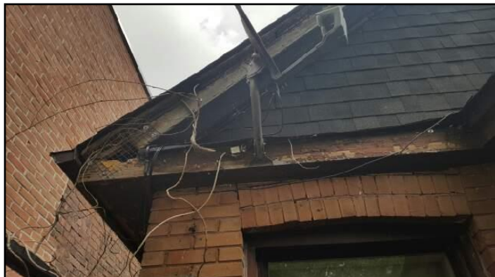
4. Paint or stain needed
