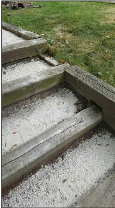
14. Rot or insect damage
