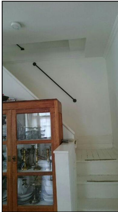
20. Missing guardrail
