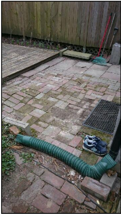
10. Poor drainage
