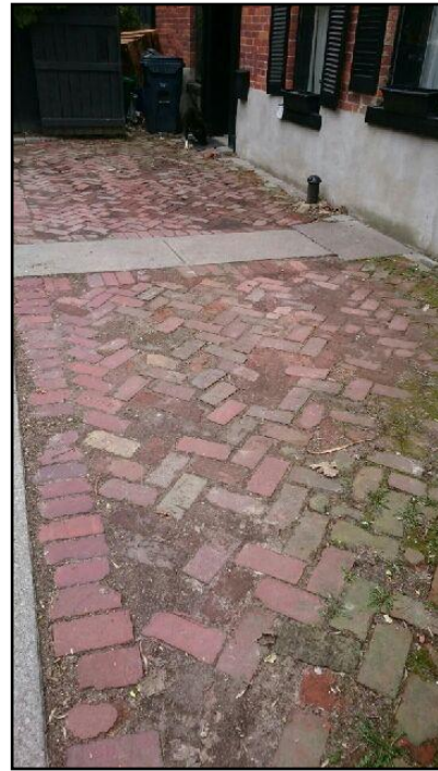
11. Poor drainage
