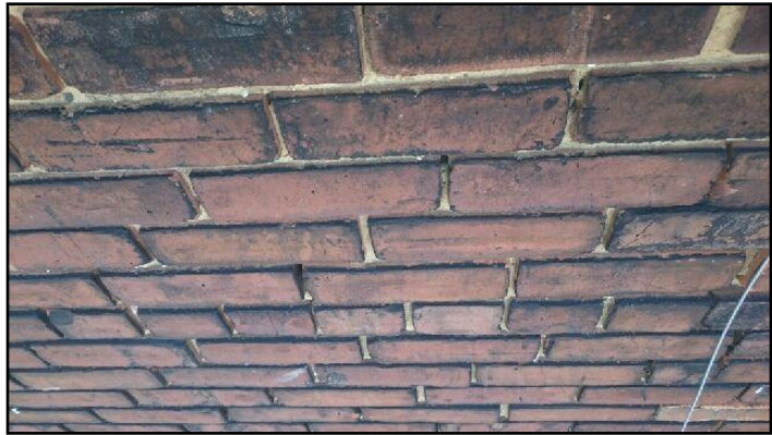
5. Mortar deterioration
