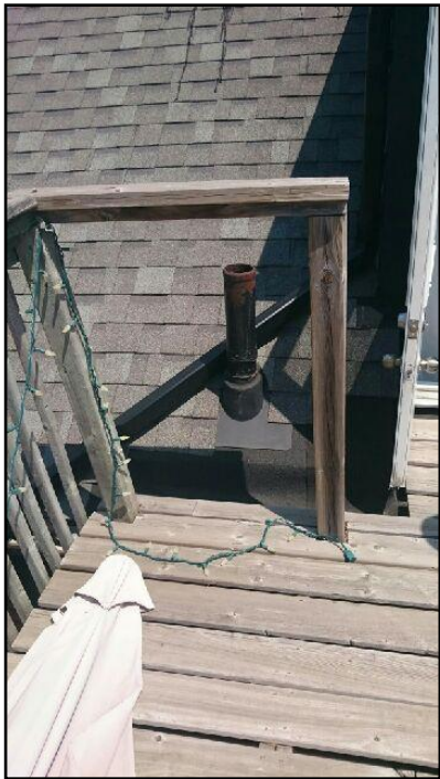
6. Missing guardrail
