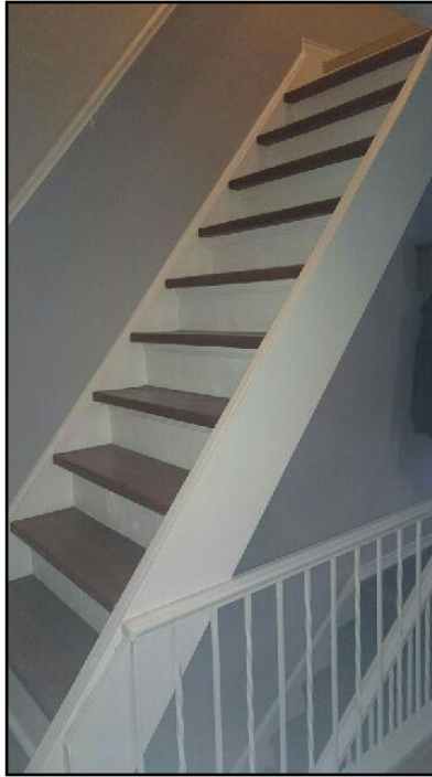
14. Missing guardrail
