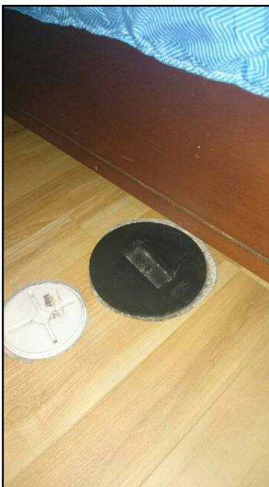
10. Present. These valves help prevent sewer...
