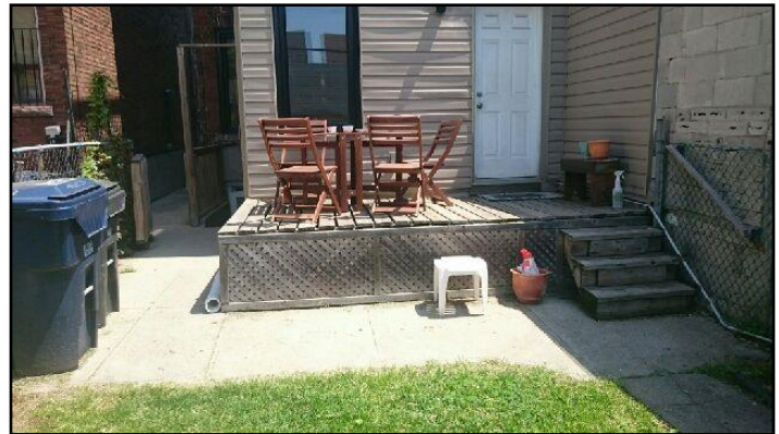
7. Missing guardrail
