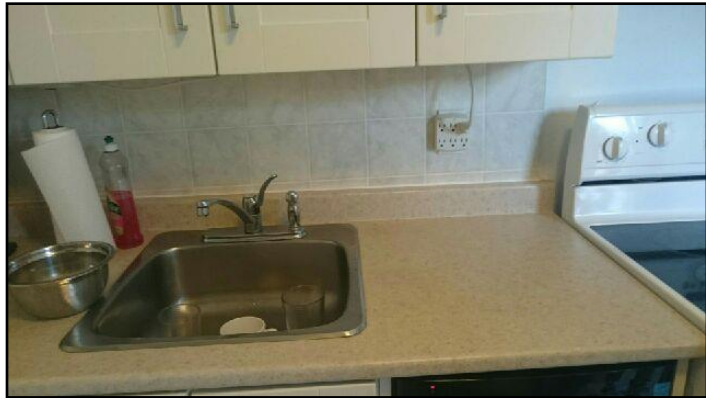
8. No GFCI (Ground Fault Circuit Interrupter)
