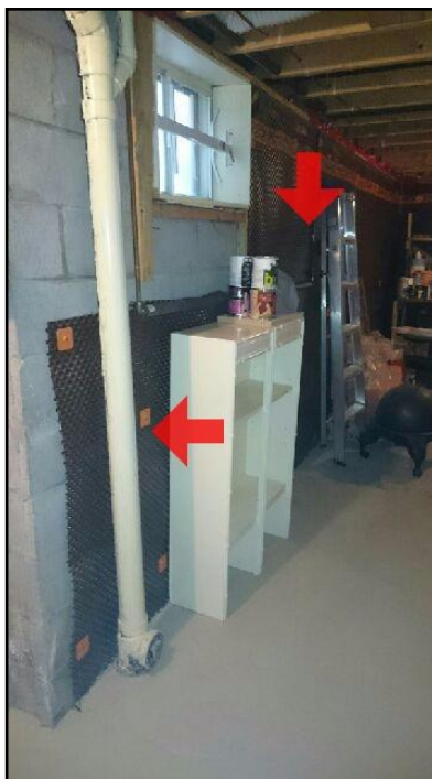
9. Interior drainage membrane.
