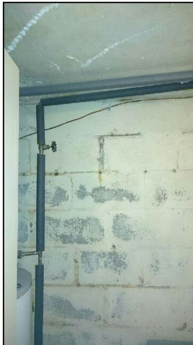
8. Efflorescence
