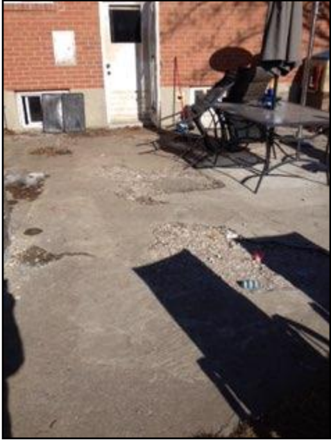
6. Concrete spalled
