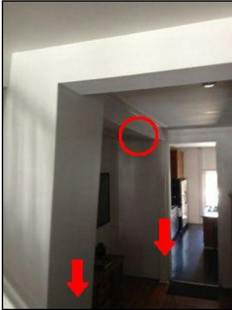
9. Support at first floor
