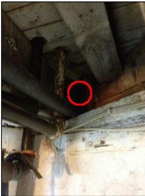
16. Potential for pipes against exterior wall t...
